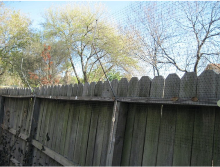
1. Bracket installed on support post
