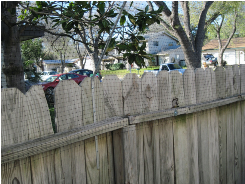
3. Bracket installed behind crossbar: tap the slat away from the crossbar and slide the bracket behind. Screw it to the wood and then tap the slat back in place. This is the way to install in snow areas.
