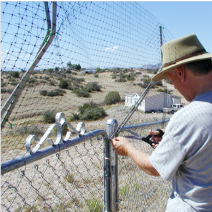
Trimming zip ties
